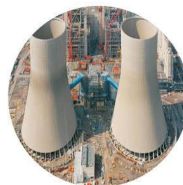
Armenia Power Plant
